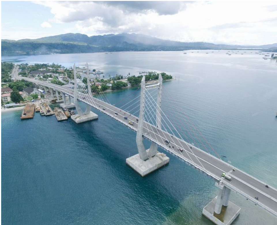
Fig. 1 Jembatan Merah Putih Cable-stayed bridge (Kementerian PUPR 2016)
